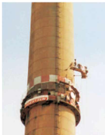
Paint removal of obsolete signage on 200 m high chimney with water-sandblasting system TORNADO and high-pressure unit E 320 - even with 150 m height still 285 bar at the nozzle.
