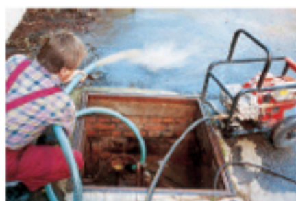
Draining of underground shaft with sludge pump - high-pressure water transports sludge away rapidly.
