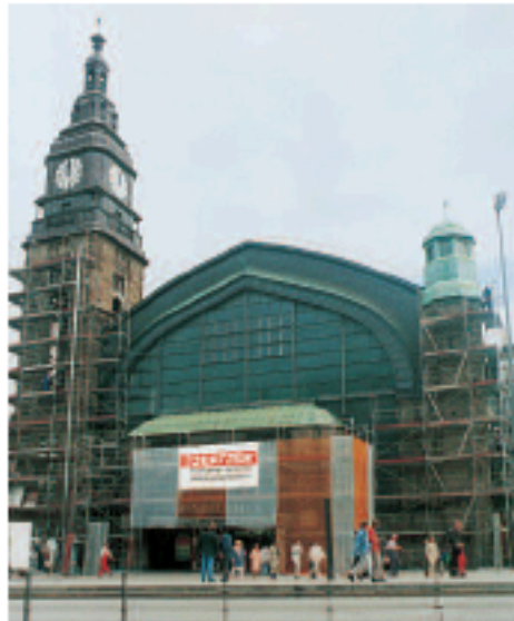
OERTZEN technology cleans sandstone facades of Hamburg central railway station
